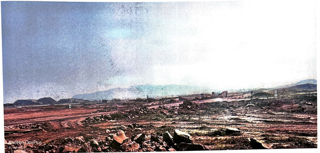
Figure 7: Runway Site before clearing the ground
