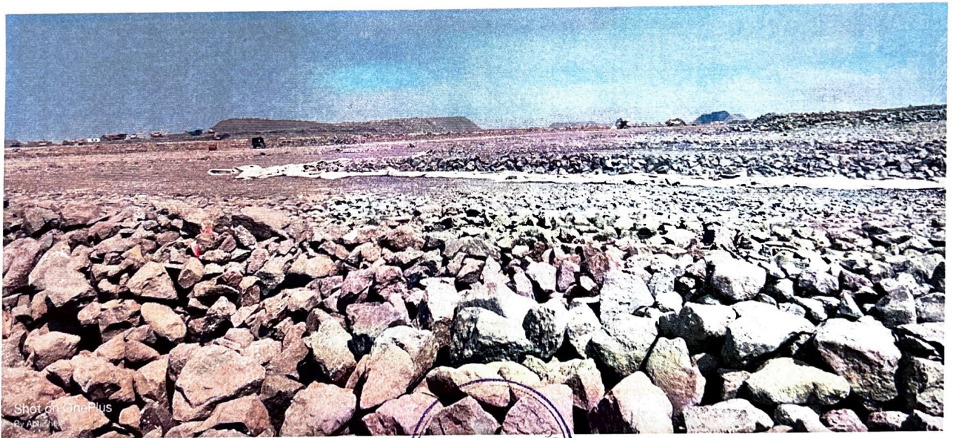
Figure 10: Local material used in the construction of the runway
